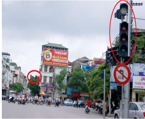
Old & broke signal
