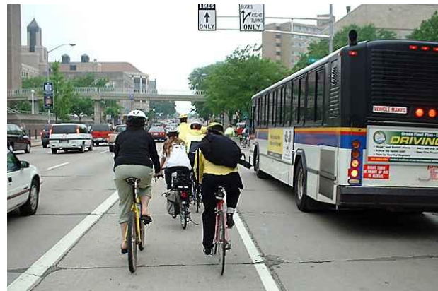
Fig. 1 Bike lane on street side of bus lane (University Ave., Madison, Wisconsin, USA.)
